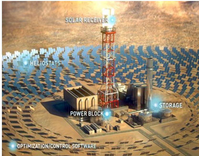
6.10 Solar Energy---Use of Melted Salt. Molten salt keeps solar power flowing. Reproduced with thanks from: http://www.cnet.com/news/molten-salt-keeps-solar-power-flowing/
